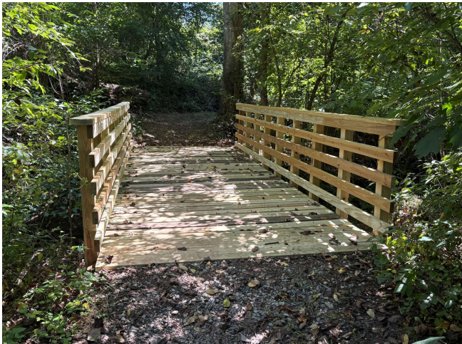
Grove – Bridge repair
