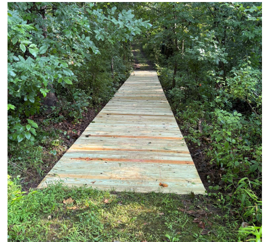
Grange – Boardwalk redecking
