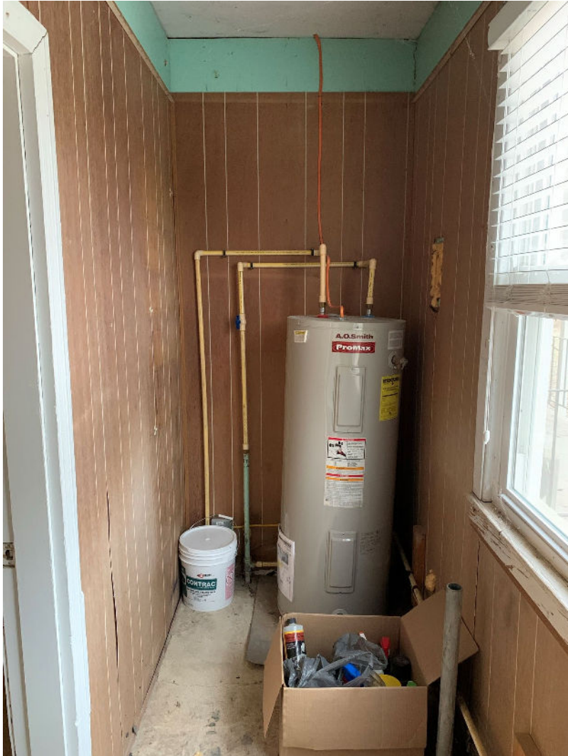
Water Closet - Before
